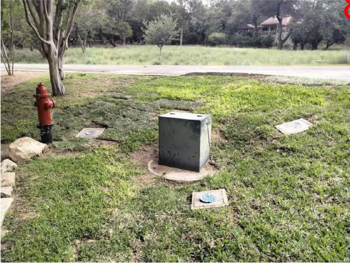
2024.05.16, Fire Hydrant & Valve Replacement at Lakeland Dr / Lakepoint Cir
