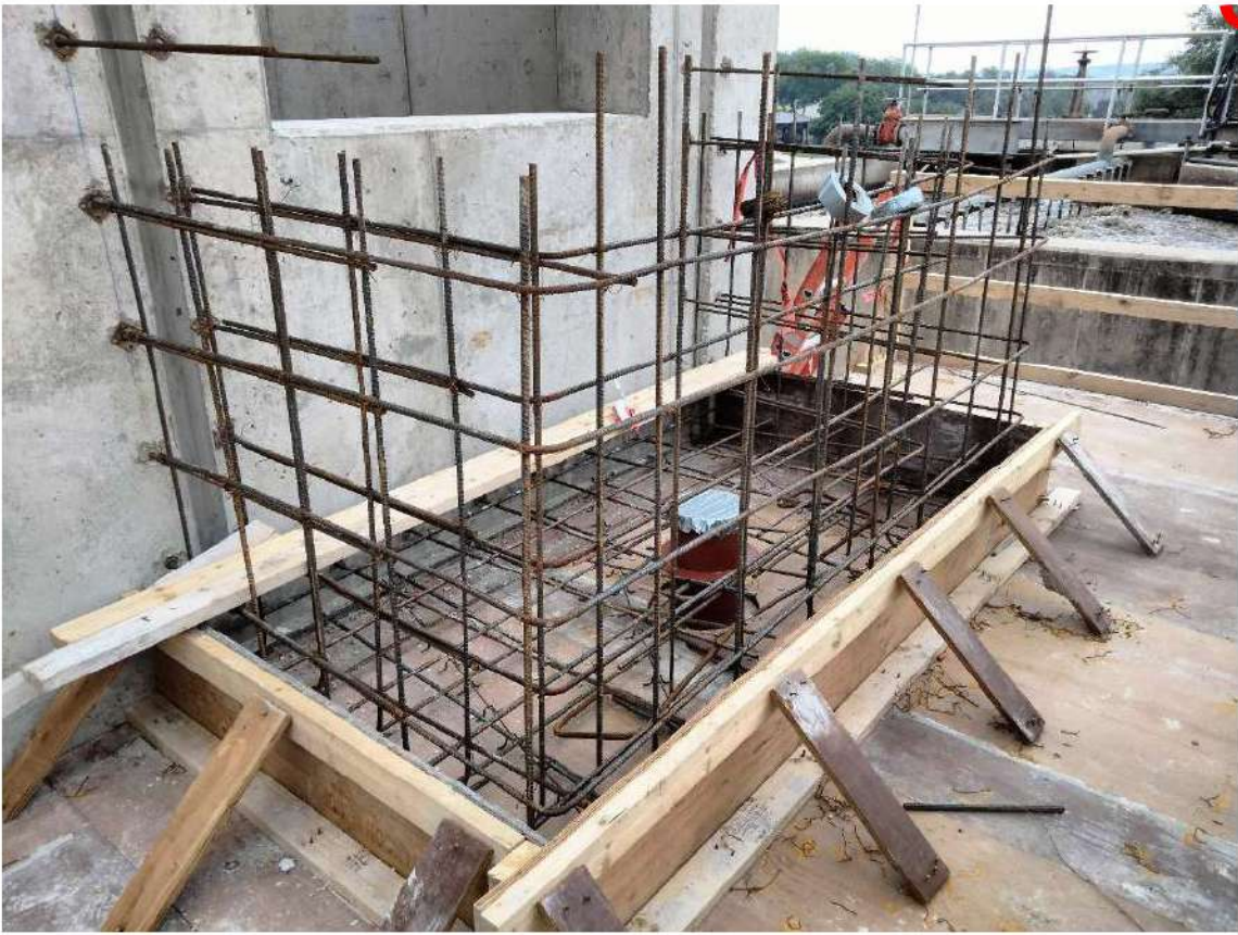
2024.05.06, Aeration Dropbox Slab Formwork & Rebar Installation
