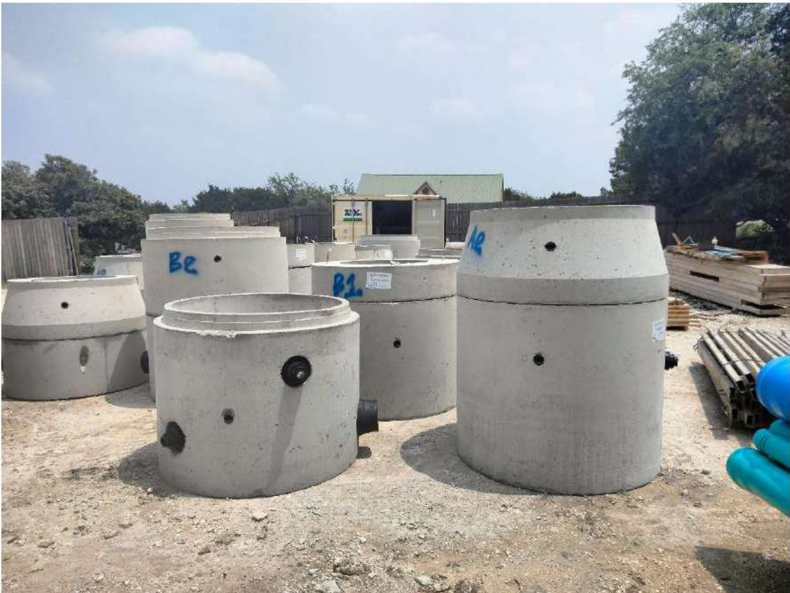
2024.05.08, Concrete Manholes Delivery
