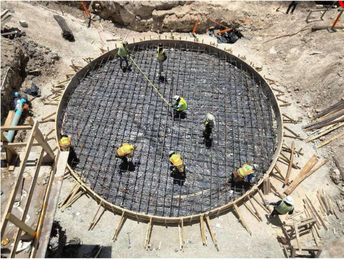
2024.05.15, Clarifier Foundation Formwork & Rebar Installation
