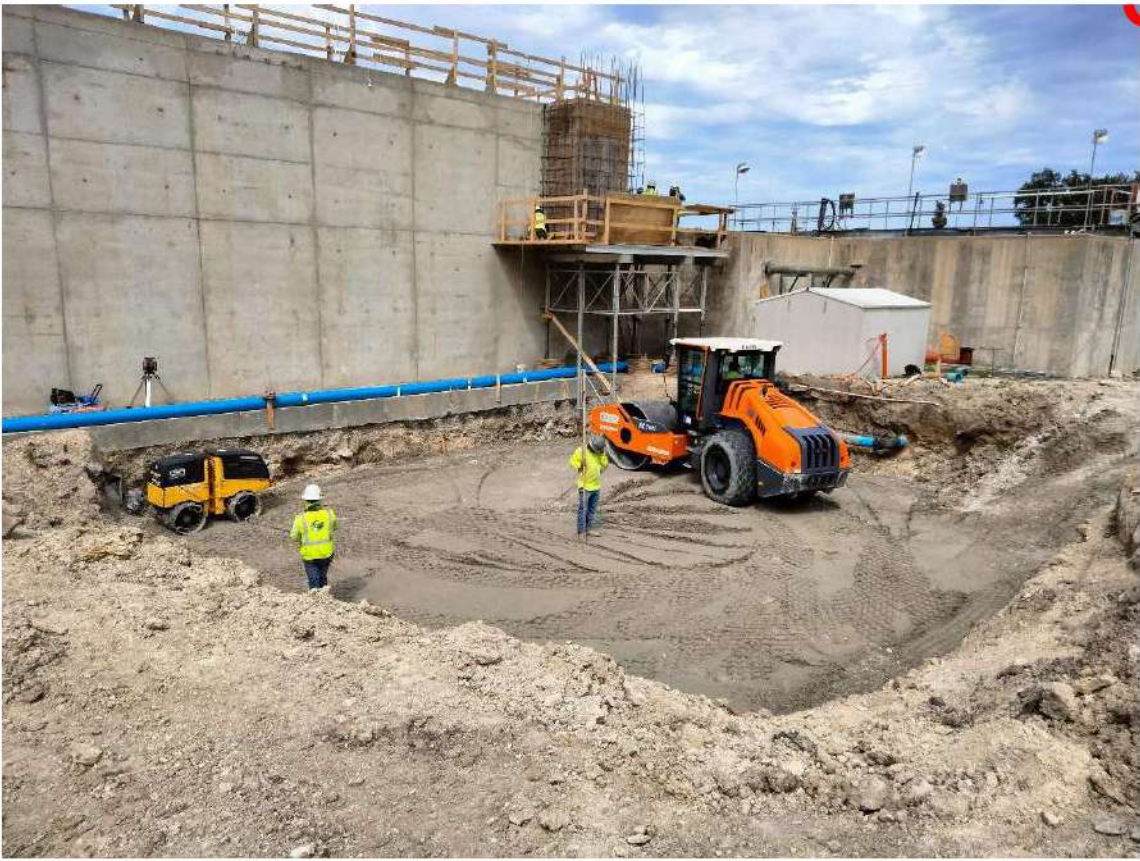
2024.05.10, Clarifier 2nd Flex Base Lift Compaction & Elevation Measurements
