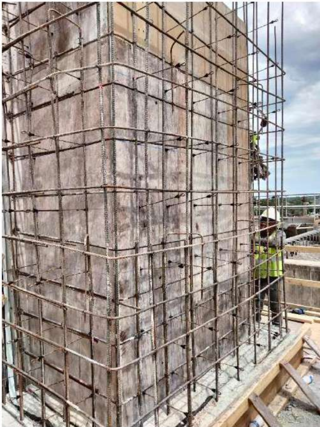
2024.05.10, Aeration Dropbox Walls Formwork & Rebar Installation
