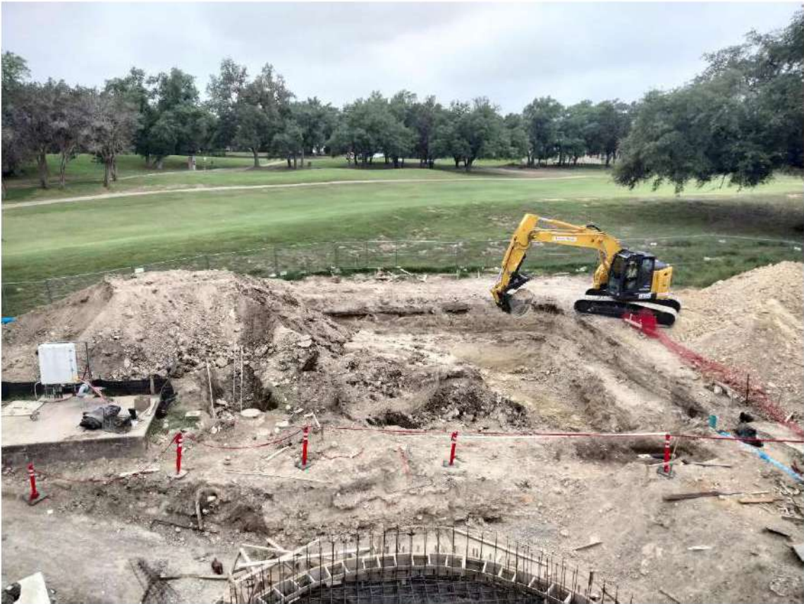
2024.05.16, Lift Station Wet Well Excavation
