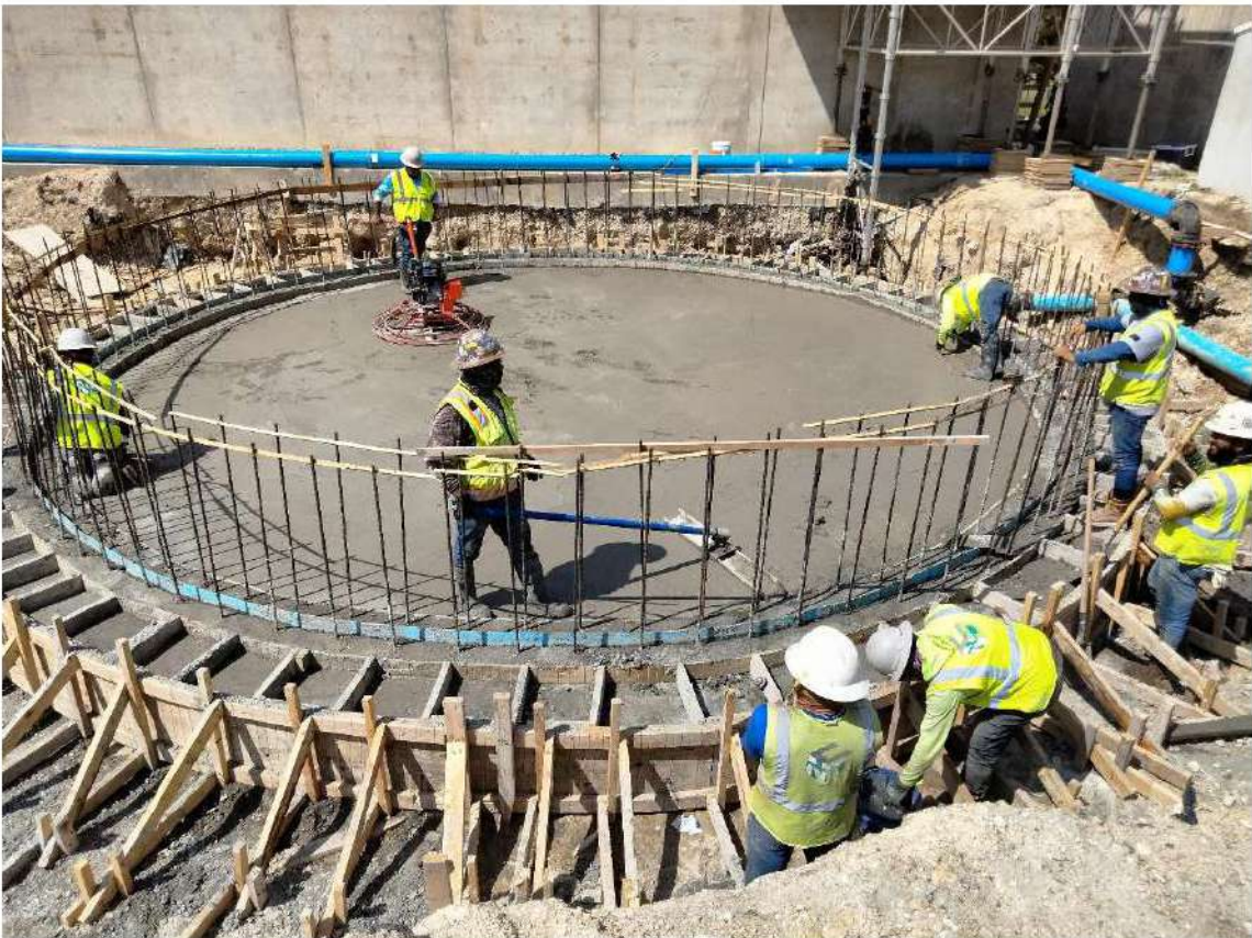
2024.05.20, Clarifier Foundation Screeding & Troweling
