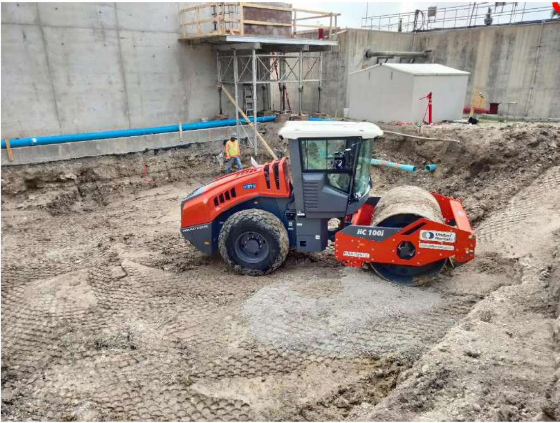
2024.05.09, Proof-Rolling Clarifier Subgrade
