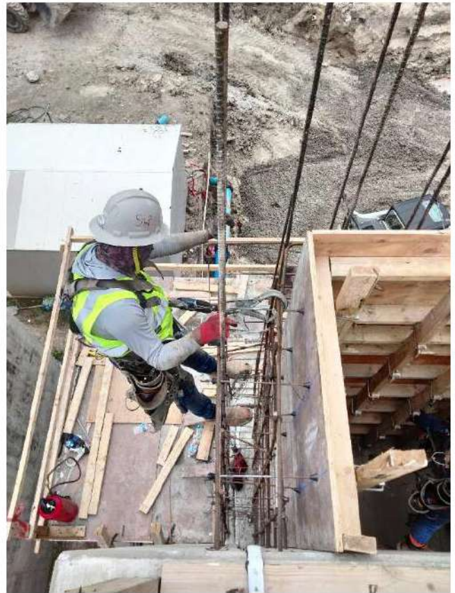
2024.05.10, Aeration Dropbox Walls Formwork & Rebar Installation
