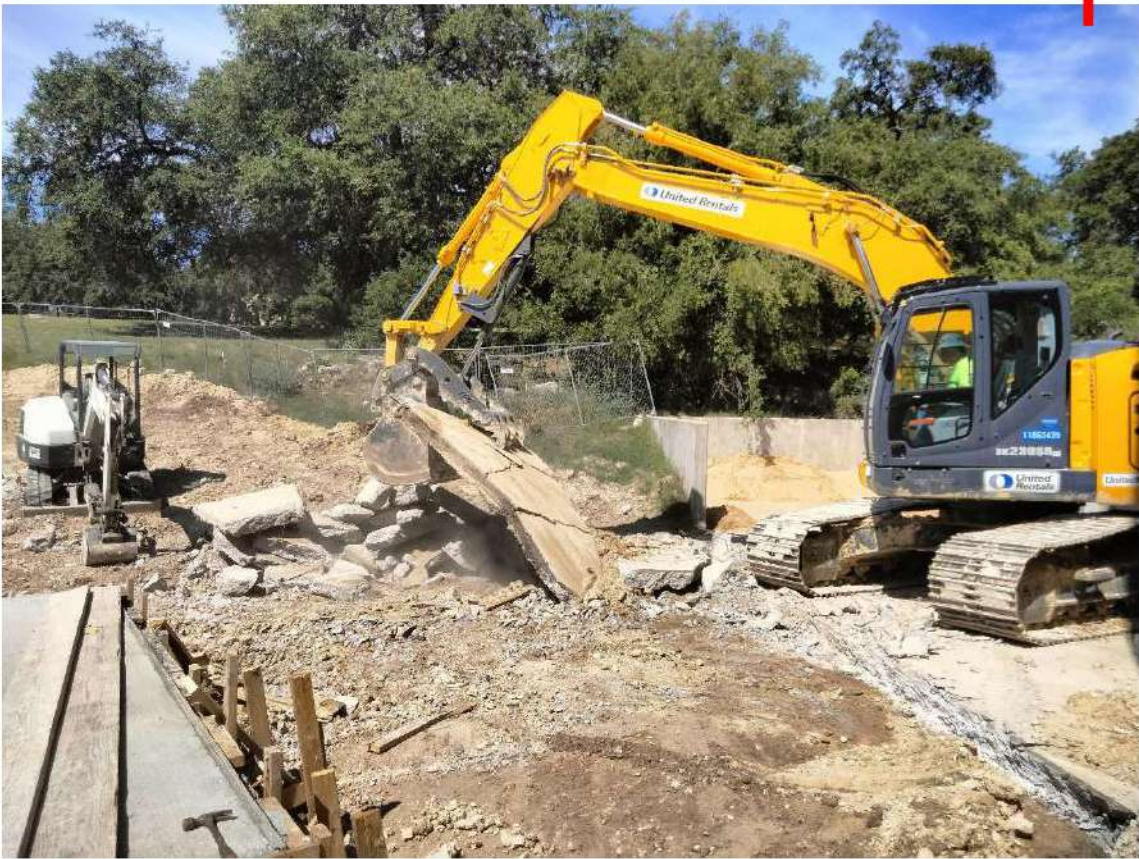
2024.06.27, Removing Section of Concrete Driveway
