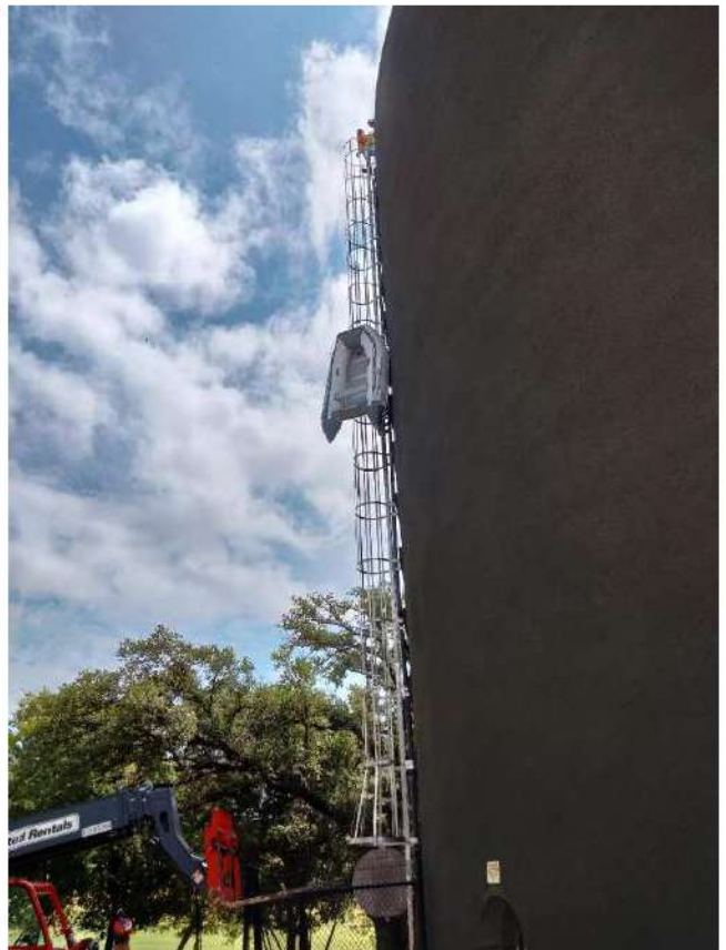
2024.07.18, Hoisting Inflatable Rafts up over top of Effluent Concrete GST
