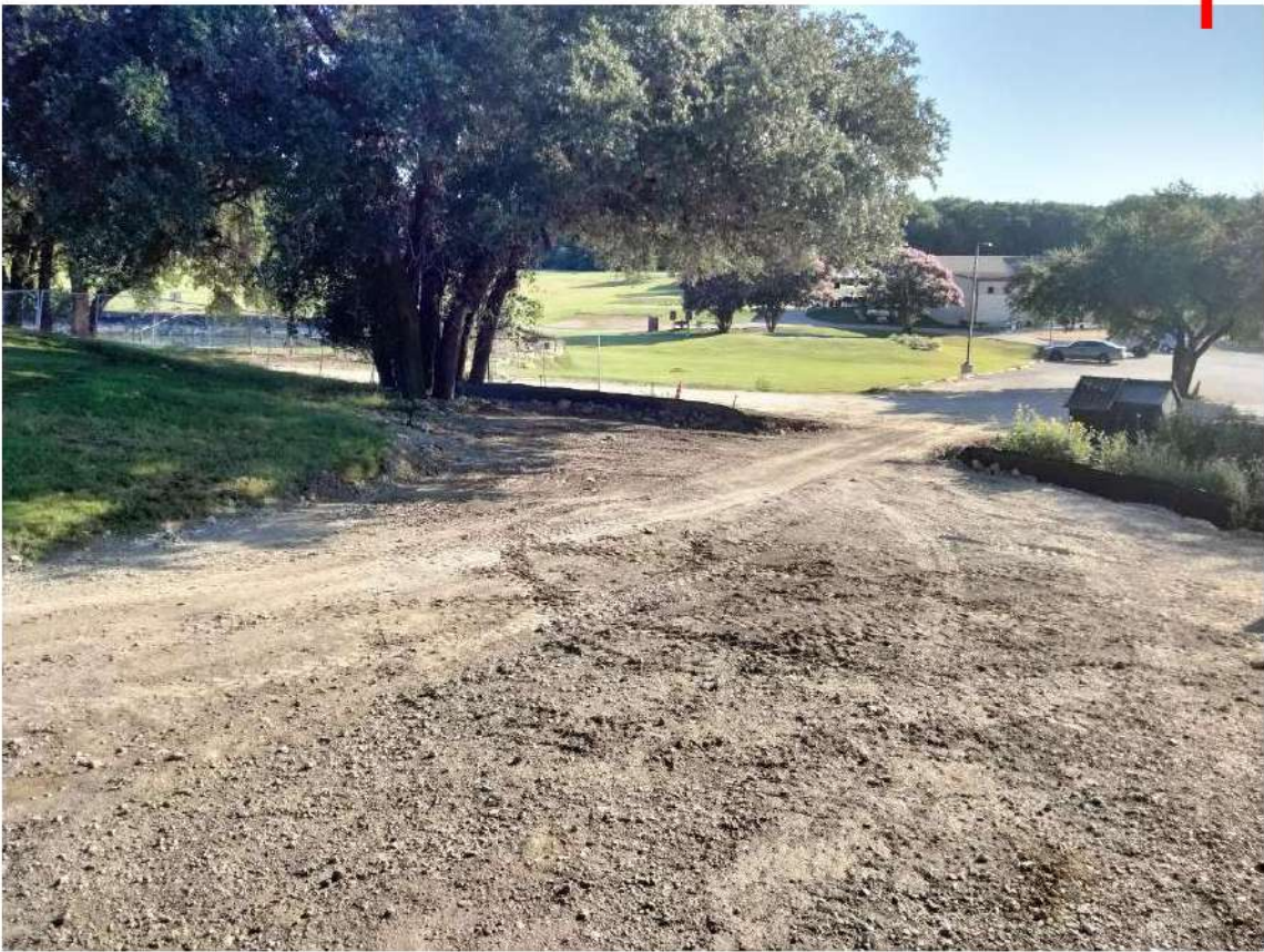
2024.07.10, Restored Entrance Prior to Construction Trailers
