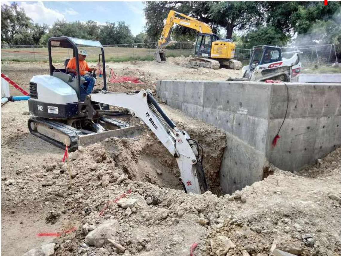
2024.07.11, Excavating for Manhole C1
