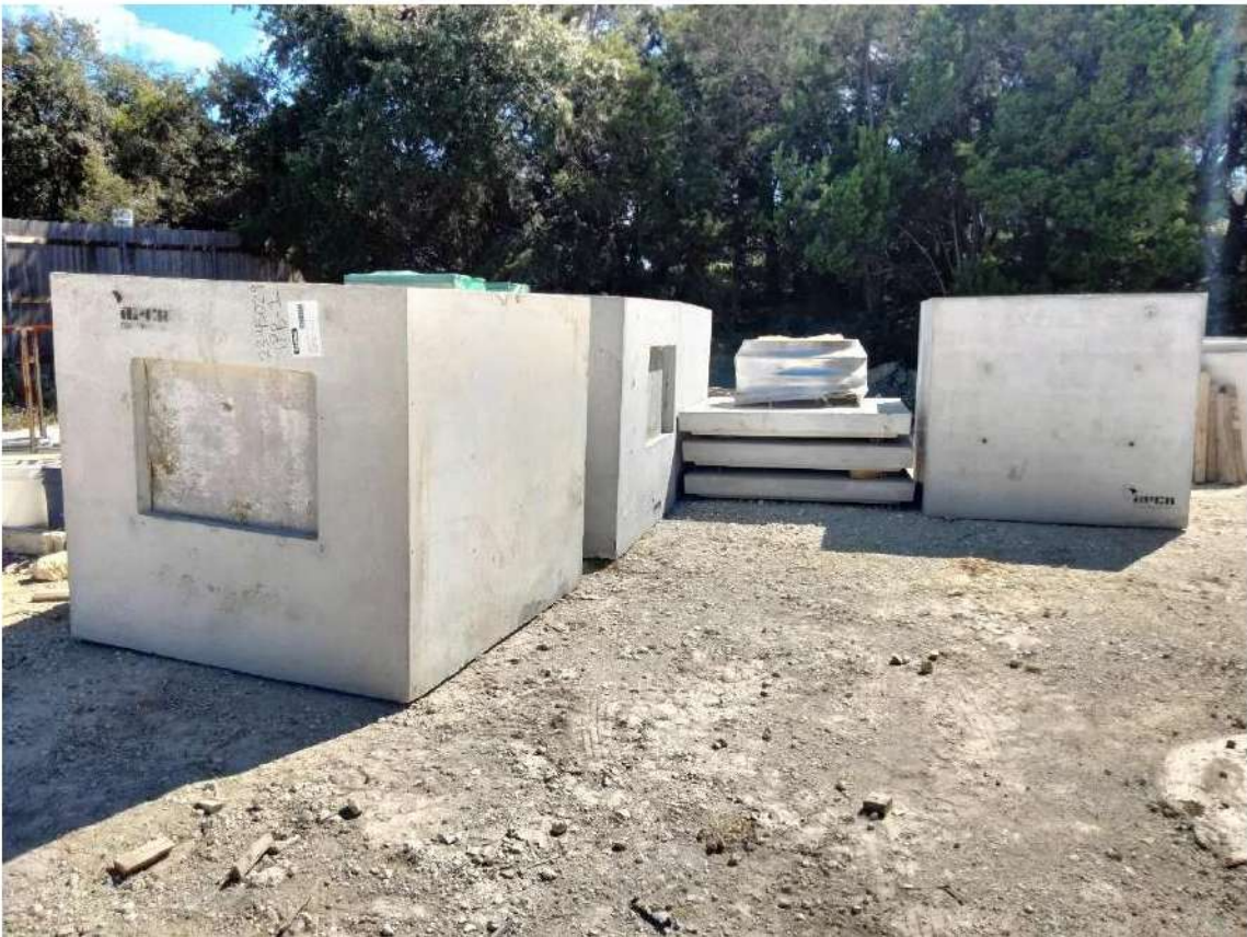
2024.09.09, Delivery of Pre-Cast Electrical Pull Boxes
