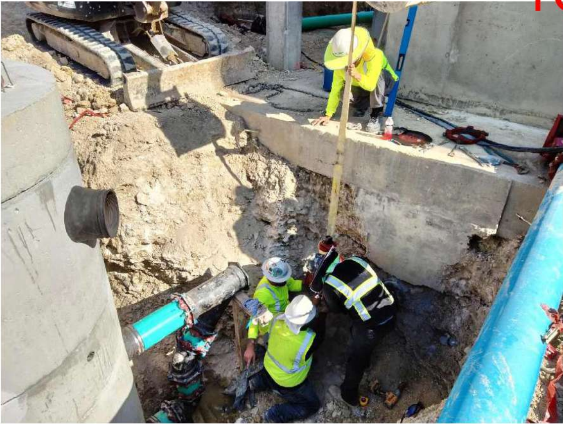
2024.09.16, Installing Gate Valve on 8" Aeration Drain Line
