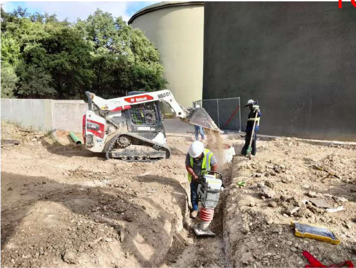
2024.08.29, Compacting Pipe Trench for 8" Gravity Main between Manholes A3 & A4
