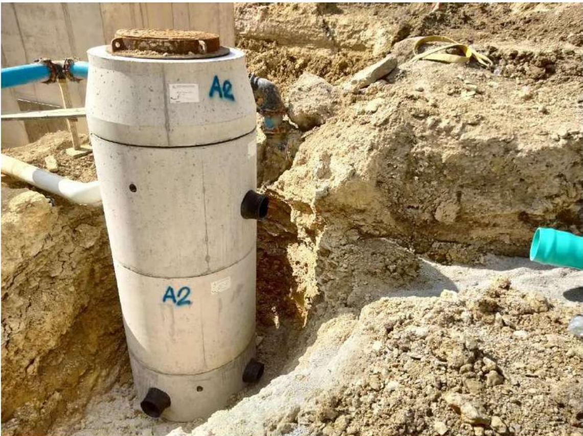
2024.09.19, Installation of Manhole A2
