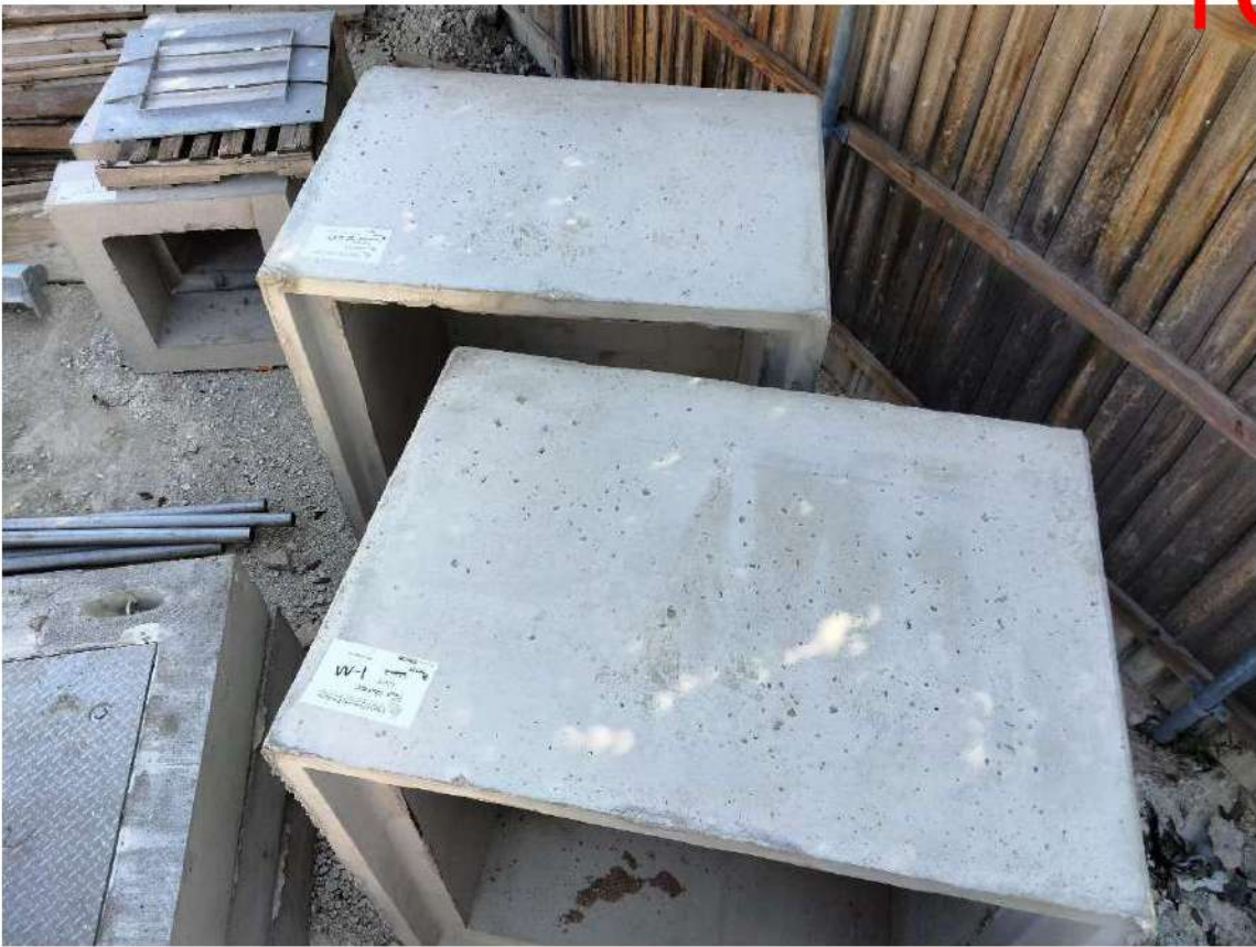
2024.09.12, Delivery of Pre-Cast Valve Vaults
