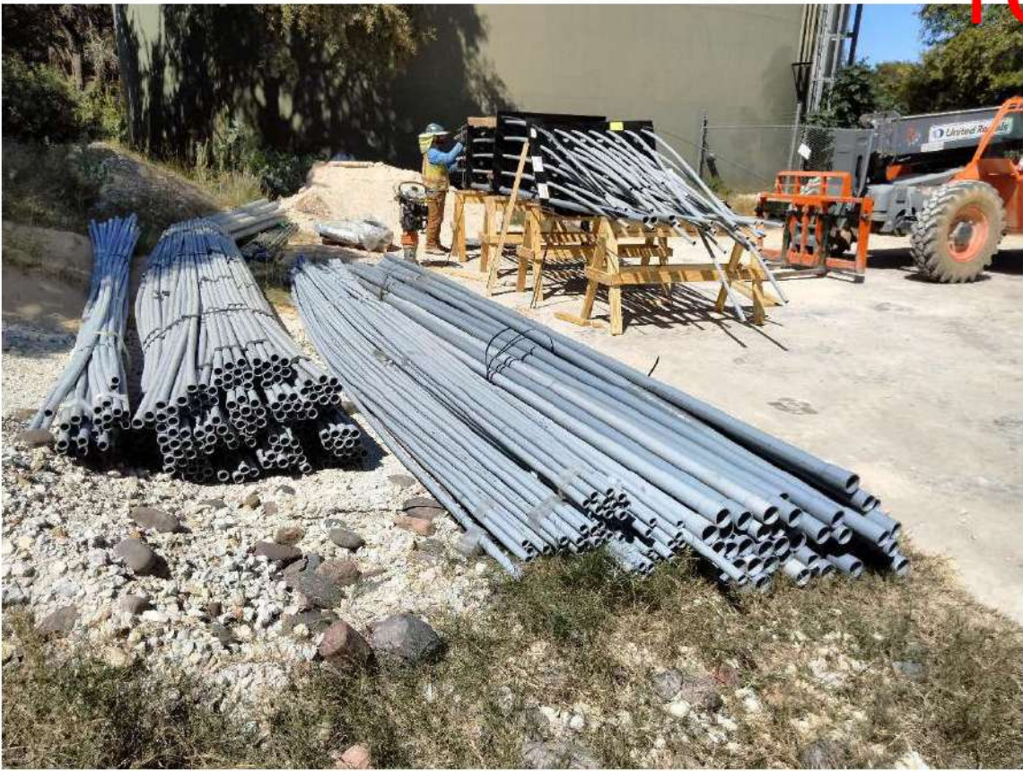
2024.10.01, Alterman Assembling Conduits for Ductbanks
