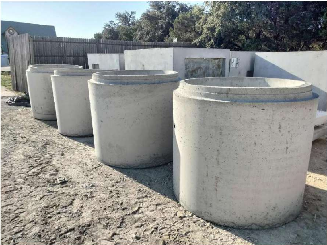
2024.10.02, Delivery of POA Lift Station Wet Well
