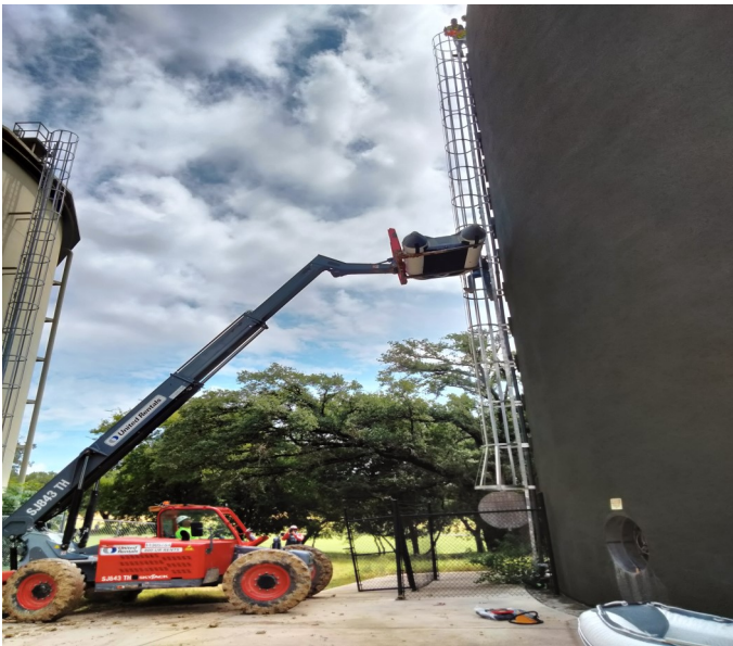
2024.07.18 - Hoisting Inflatable Rafts up over top of Effluent Concrete GST
