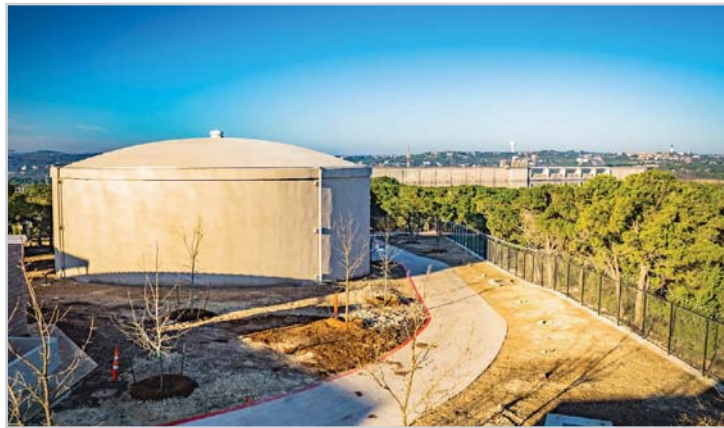
Mansfield WTP Clearwell Nos. 1 Elevated Storage Tank
