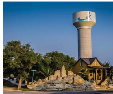
Mountain View Elevated Storage Tank
