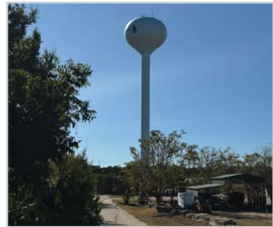
Hudson Bend Elevated Storage Tank
