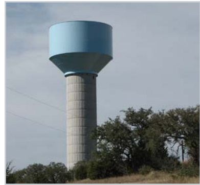
Highway 71 Elevated Storage Tank
