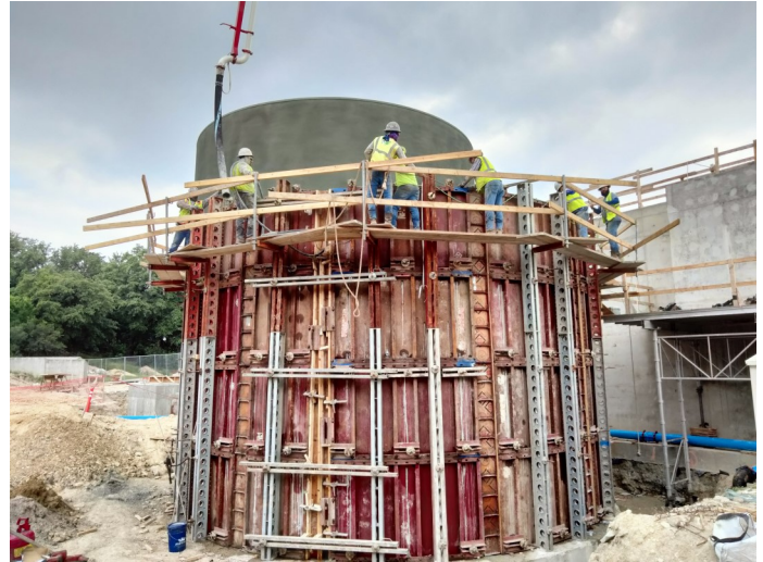
2024-06-03 - Clarifier Wall Concrete
