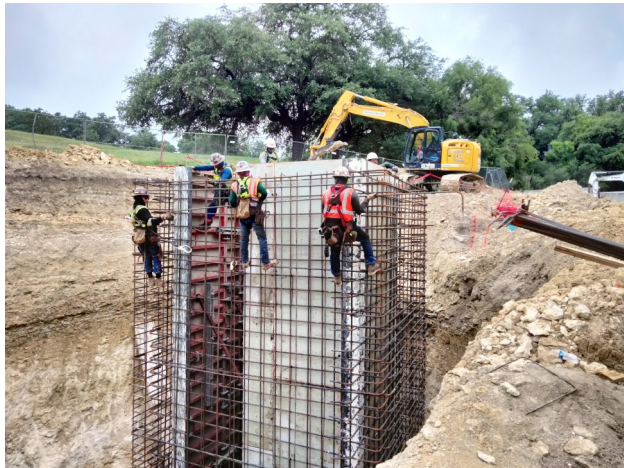
2024-06-12 Wet Well Walls Rebar Installation
