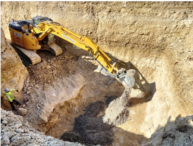
2024-06-06 Wet Well Foundation Flex Base Installation
