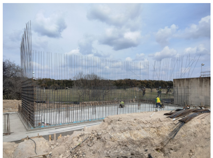
Headworks/aeration basin for new WWTP.
