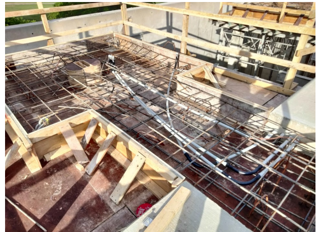
04.10.24, West Aerator Platform Formwork & Rebar Installation
