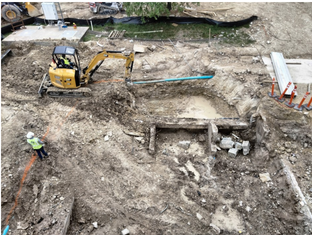
04.10.24, Excavation for Clarifier
