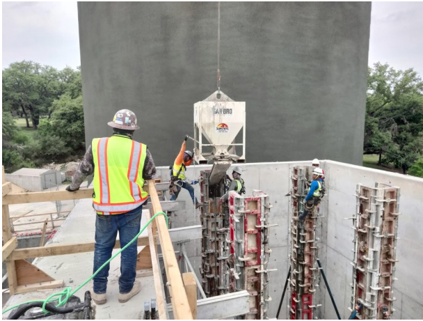
4-1-24, concrete pour for the interior aeration basin columns via concrete bucket
