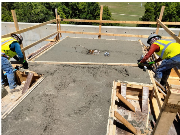
4.11.24, Screeding East Aerator Platform
