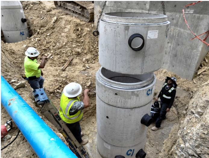
2024.09.03, Setting Manhole C1
