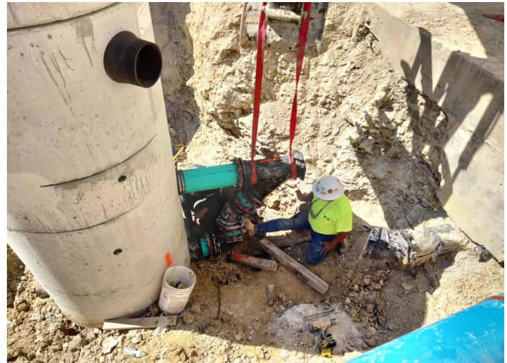
2024.09.12, Installing Drop Connection for Manhole C1
