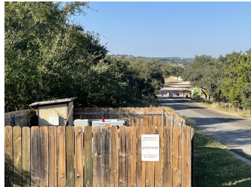
Whispering Hollow Lift Station-Be Cautious During Construction
