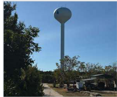
Hudson Bend Elevated Storage Tank
