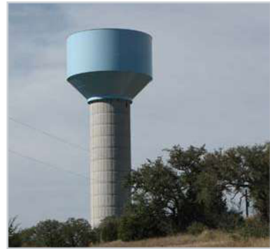
Highway 71 Elevated Storage Tank
