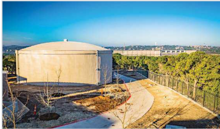
Mansfield WTP Clearwell Nos. 1 Elevated Storage Tank
