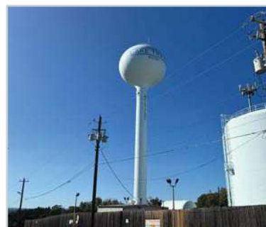
Comanche Trail Elevated Storage Tank
