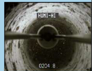
Representative well survey video stills: well wall below production zone at 205-foot depth.
