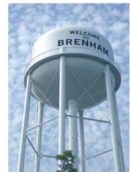
Church Street elevated water storage tank.
