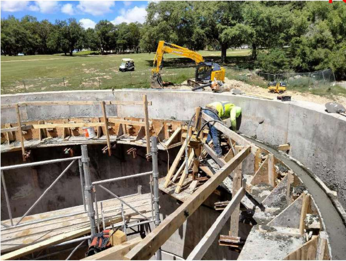
2024.06.24, Clarifier Weir/Trough Concrete Troweling
