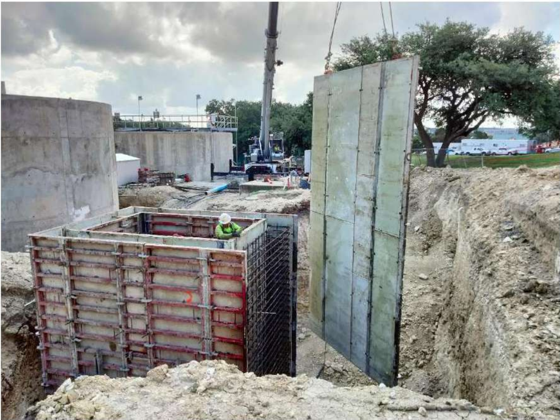
2024.06.13, Wet Well Walls Exterior Form Installation
