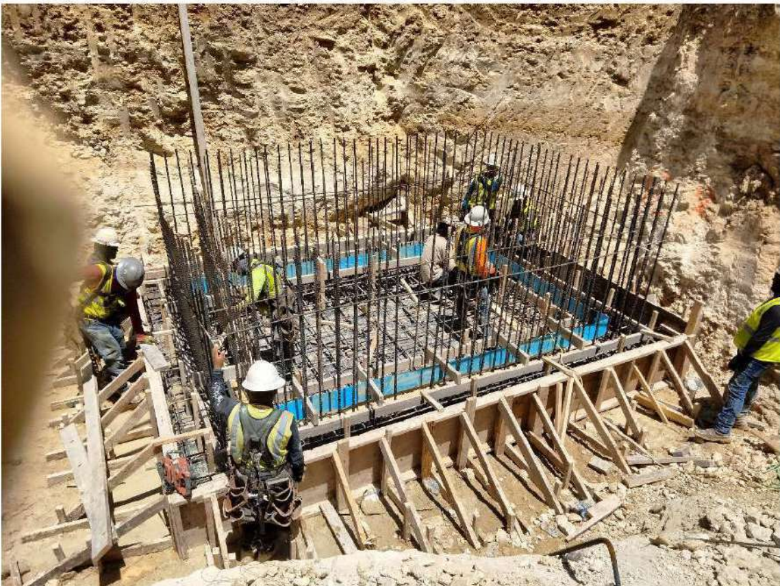
2024.06.07, Wet Well Foundation Forms & Rebar Installation
