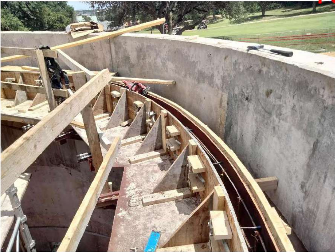
2024.06.21, Clarifier Weir/Trough Forms & Rebar Installation
