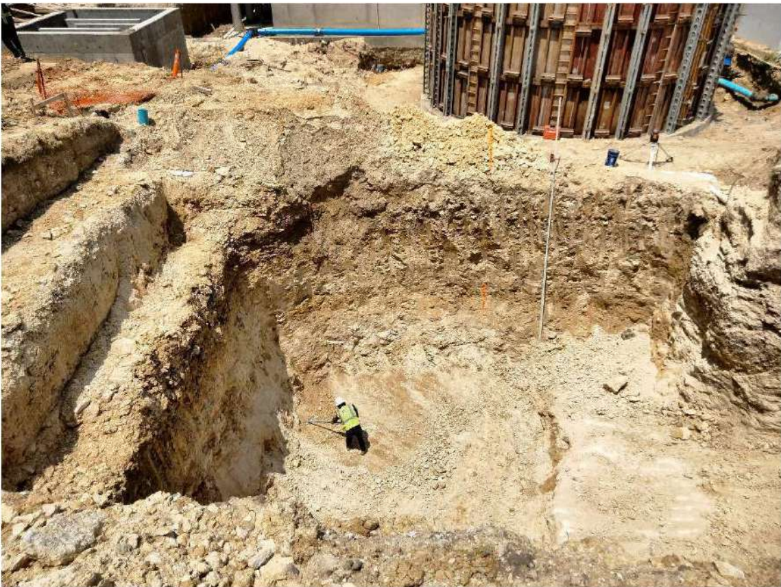
2024.06.05, Wet Well Excavation & Subgrade
