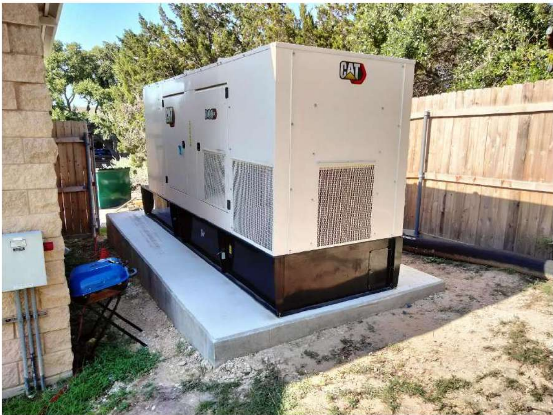
2024.06.07, GenSet & Concrete Equipment Pad
