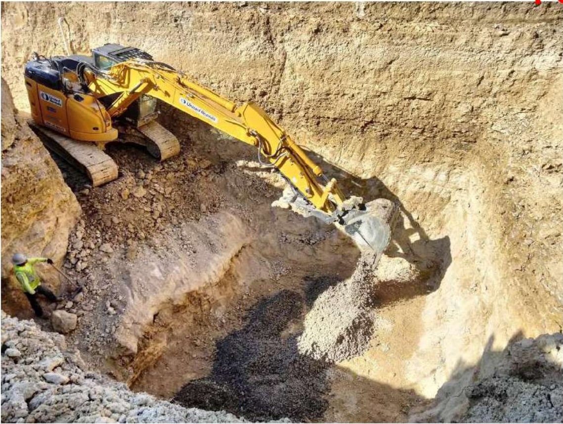
2024.06.06, Wet Well Foundation Flex Base Installation
