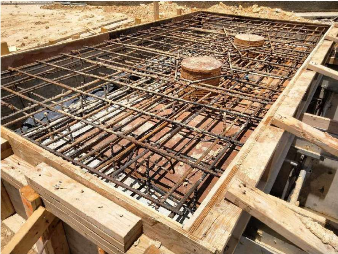
2024.06.21, Effluent Transfer Top Slab Forms & Rebar Installation
