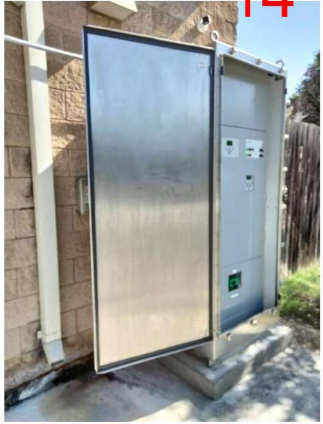
2024.06.07, Automatic Transfer Switch
