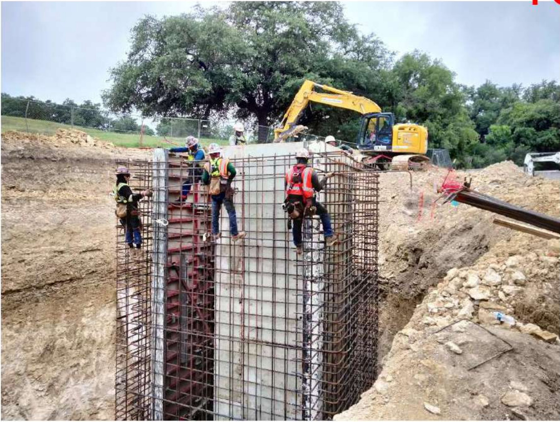
2024.06.12, Wet Well Walls Rebar Installation
