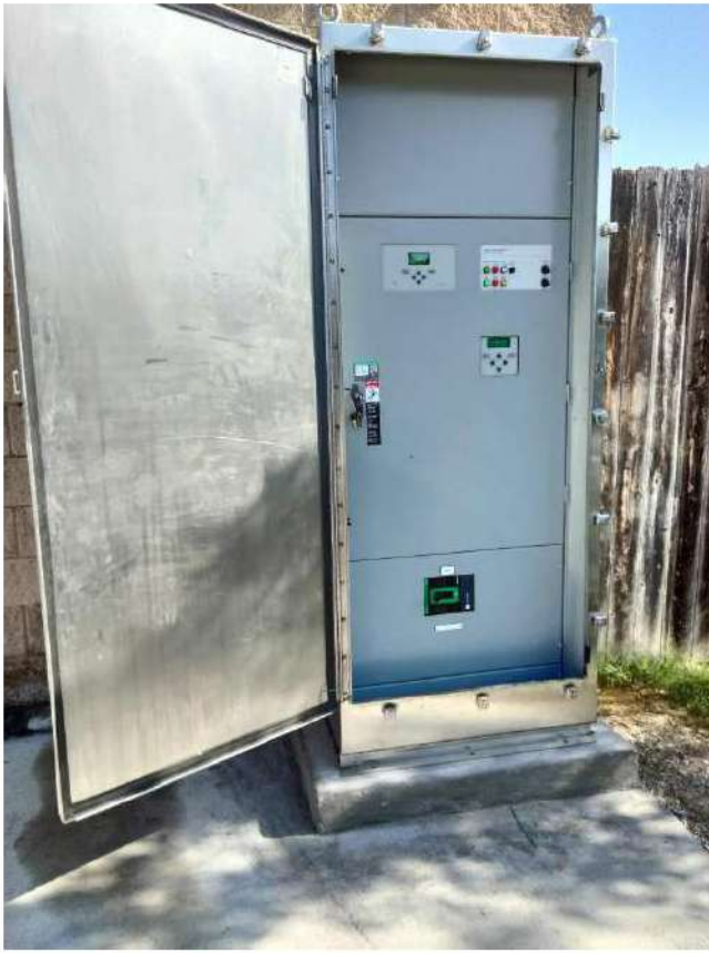
2024.06.07, Automatic Transfer Switch
